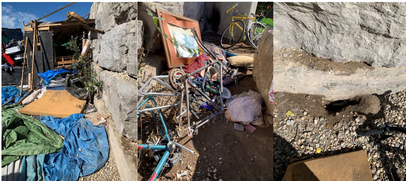
Conditions of North Rock Wall, including rodent burrow hole:
